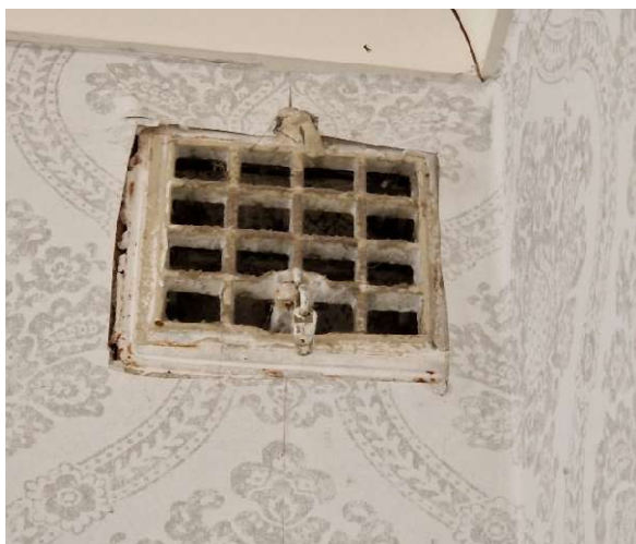
Figur 26 Ventilationsgaller.
